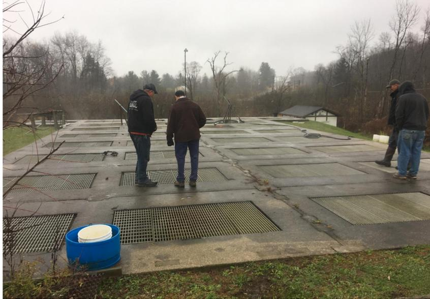
Concrete Aeration, Clarifier, and Settling Tankage
