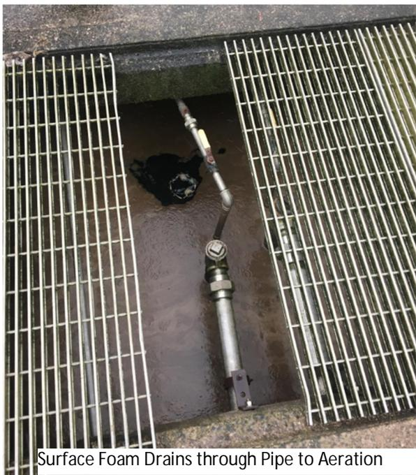
Surface Foam Drains through Pipe to Aeration
